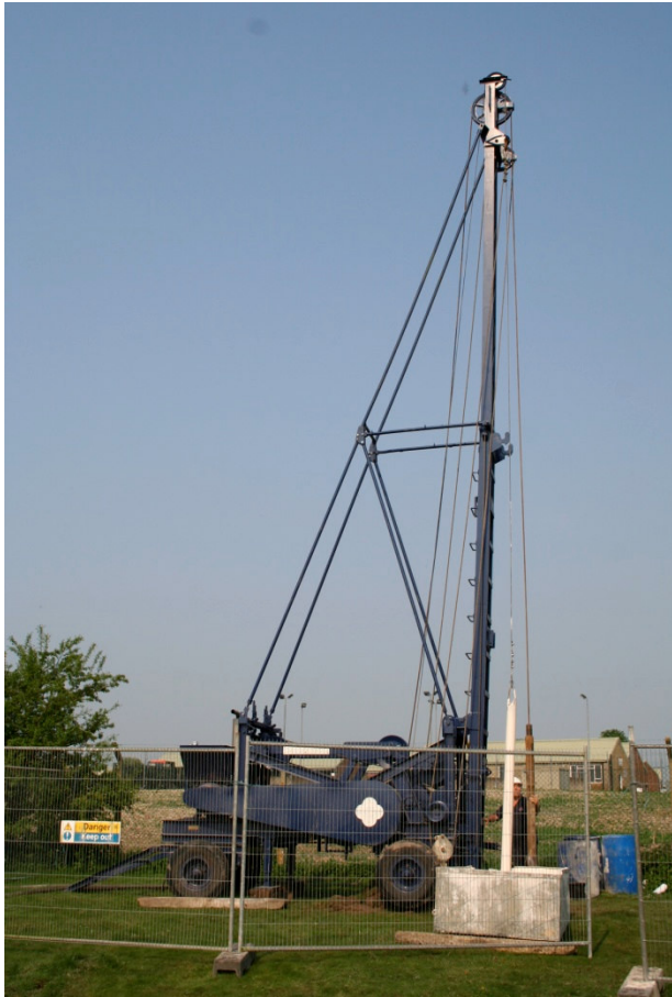
Dando 800 percussion rig drilling an observation borehole for Wessex Water.
